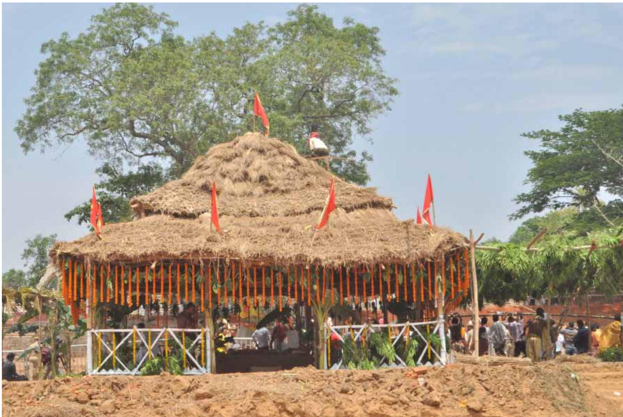
A Mandap is erected at the site of the Daru for conducting Yajna. The Sudarshan Daru is seen in the background.
